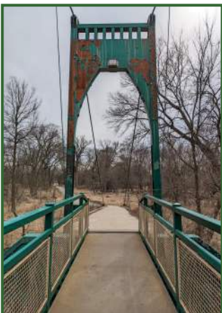
The current state of the Swinging Bridge, first erected in 1940.
